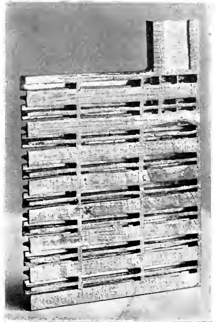
FIG. 1.—BATTERY GRID.
